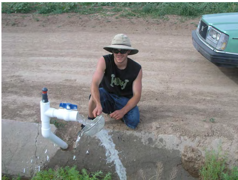
Checking flush water for particles with a strainer
