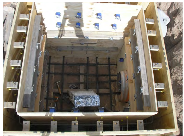
10. Rebar, forms and snap ties in place!
