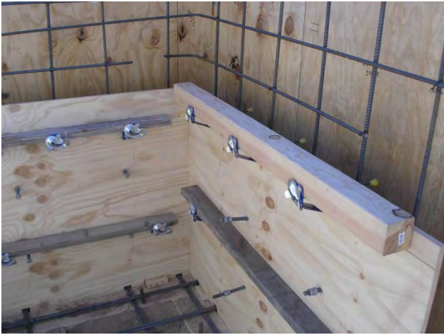
7. "Snap tie" bracing
