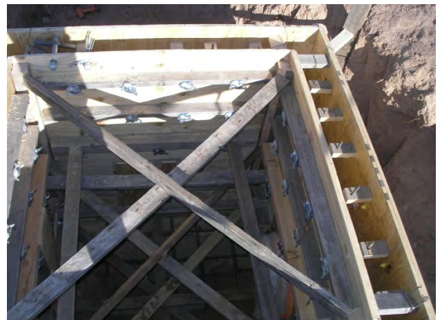
12. Internal bracing for support
