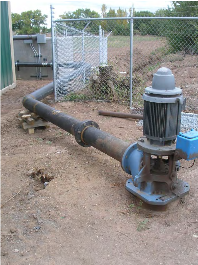
well with piping leading to concrete box "wet well"
