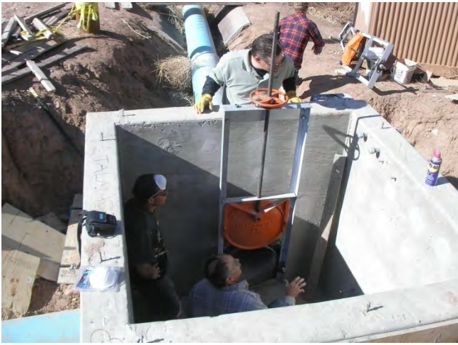
19. The canal gates go on!
