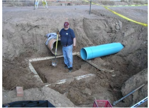
2. Outer collar in place, digging stem wall
