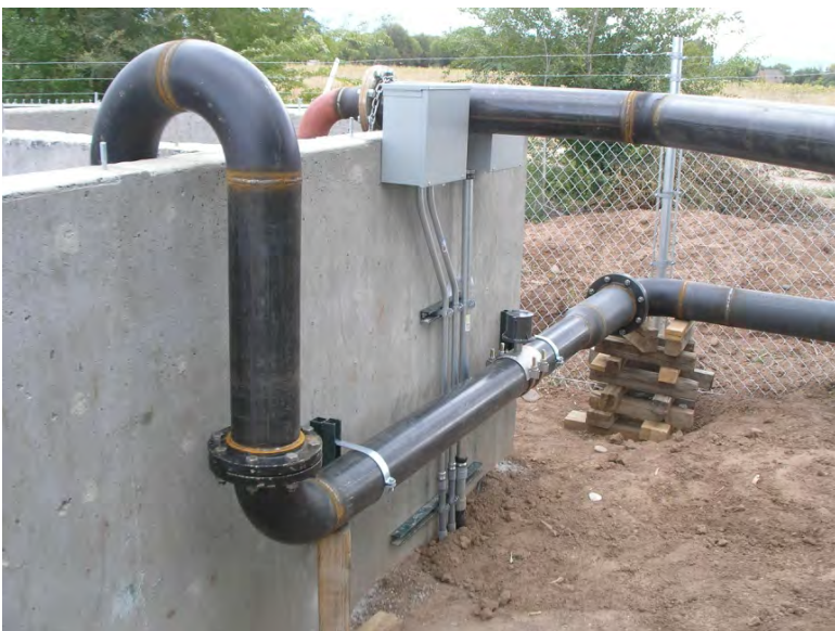
well water pumps into one side of the 2 chamber "wet well"
