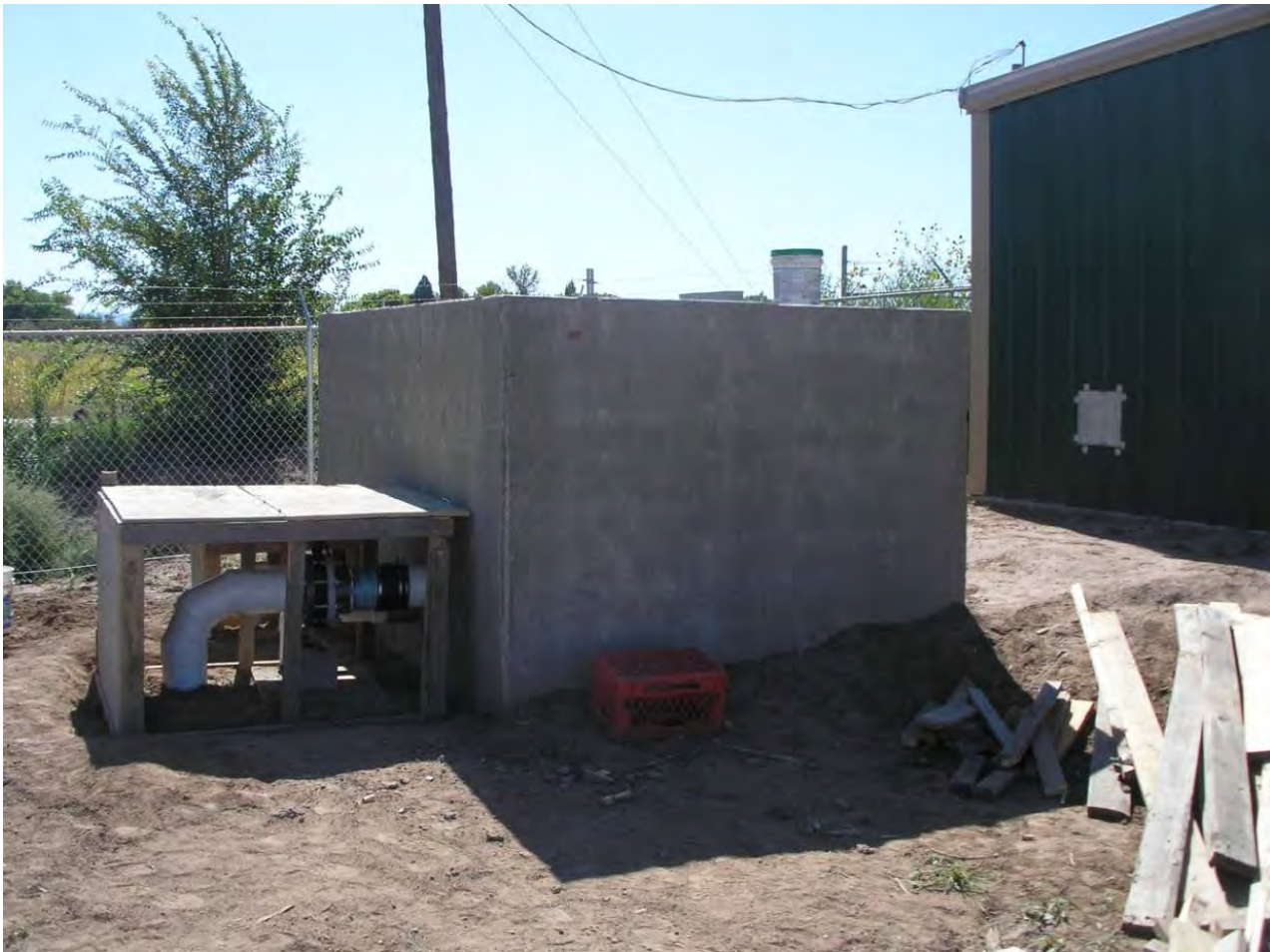
Concrete two chamber "wet well". Note surface water piping on left. Ditch water enters here and is controlled by a butterfly valve.
