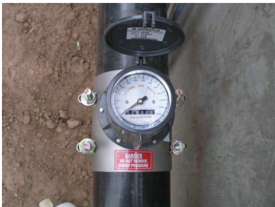
Meter used to measure well water
