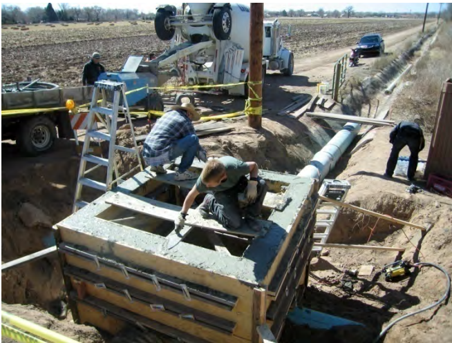
15. Finishing out the walls
