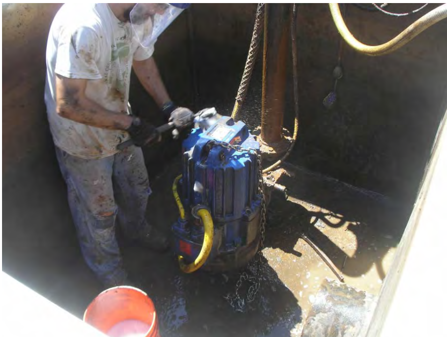
Cleaning the booster pump
