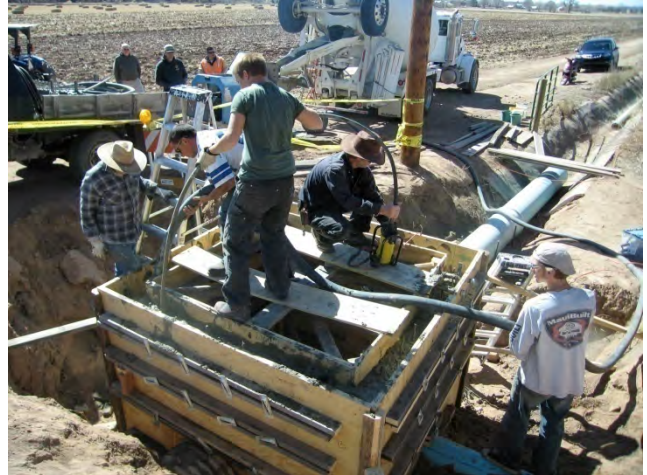
14. Concrete is pumped in and vibrated
