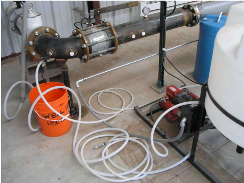
Injector pump- in red, lower right of photo
