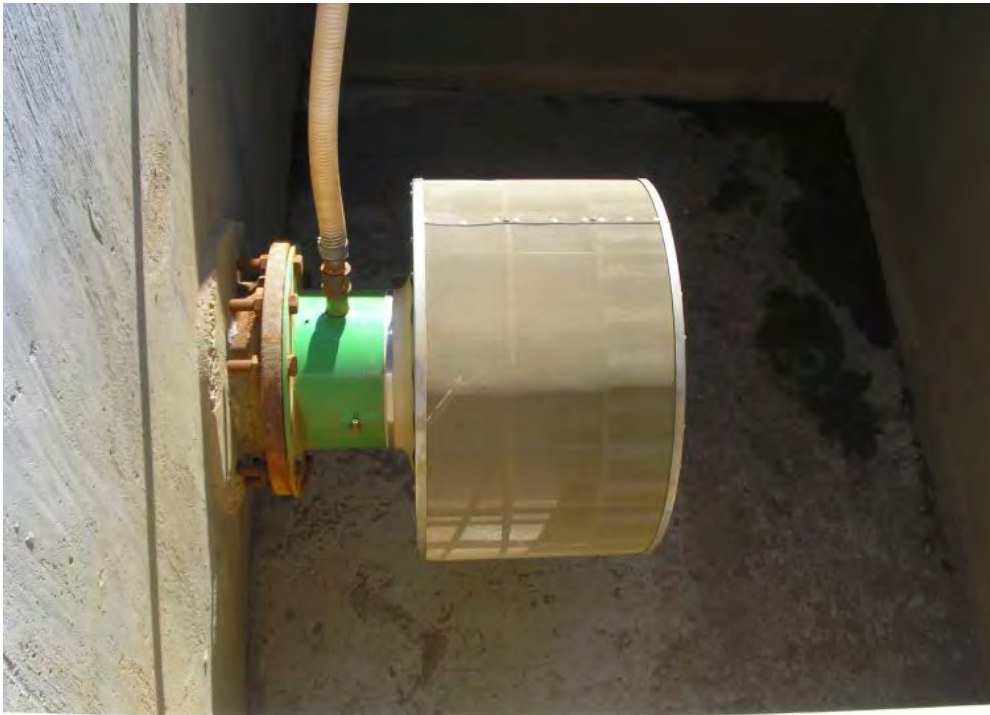
Spinner prefilter leading from chamber one to chamber two.
