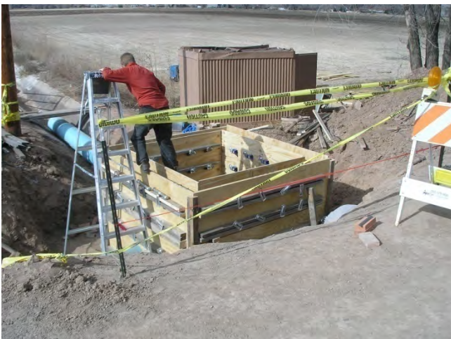
11. Note the "Jahn A" bracing system on box
