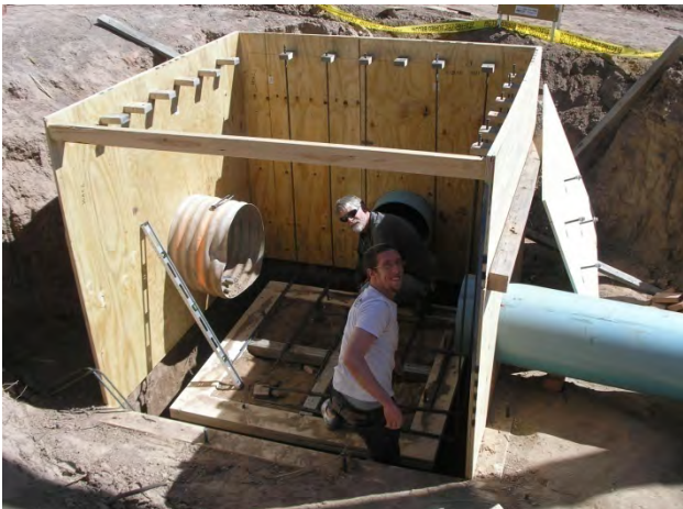
5. Inner collar is placed, 1/2" rebar goes in
