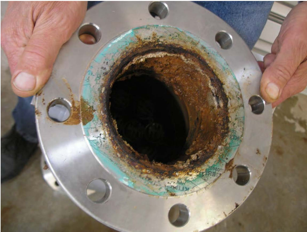
Mineral scale buildup before water treated by Zetacore unit
