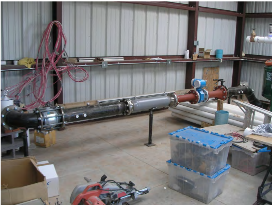
View of the main line in the wellhouse showing flow meter, Zetacore unit and pressure reducing valve
