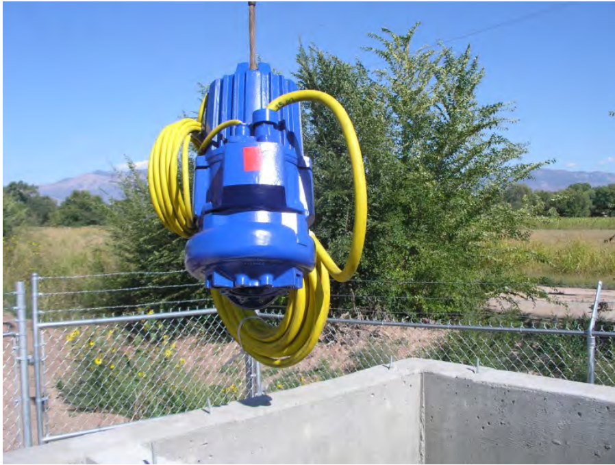
submersible pressure pump being lowered into wet well
