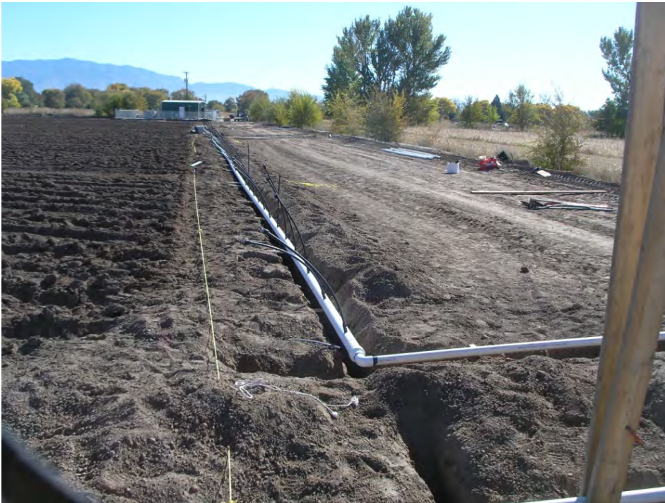
flush line manifold
