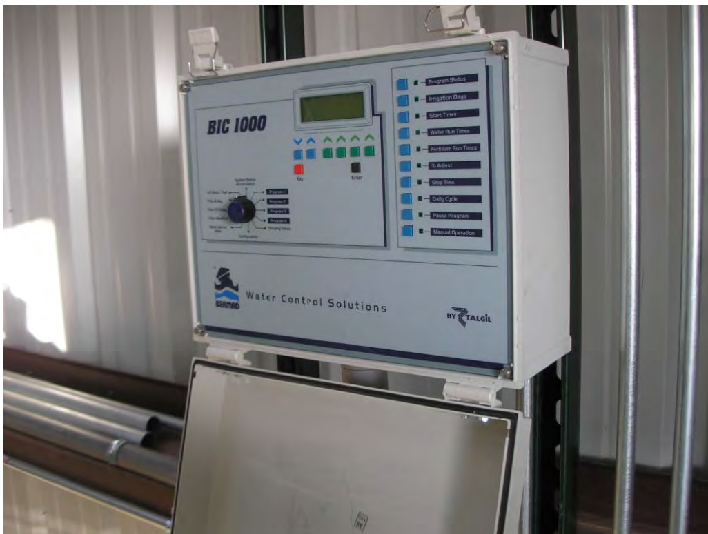
Zone valve controller- can be fully automated
