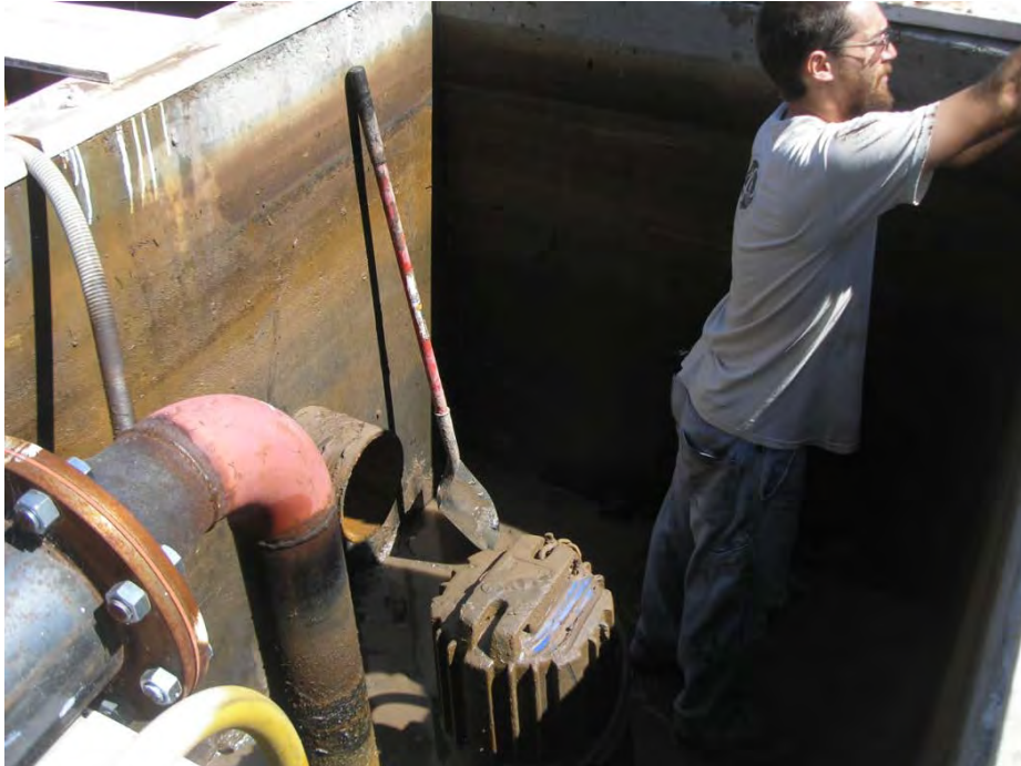
Cleaning out the water collection box
