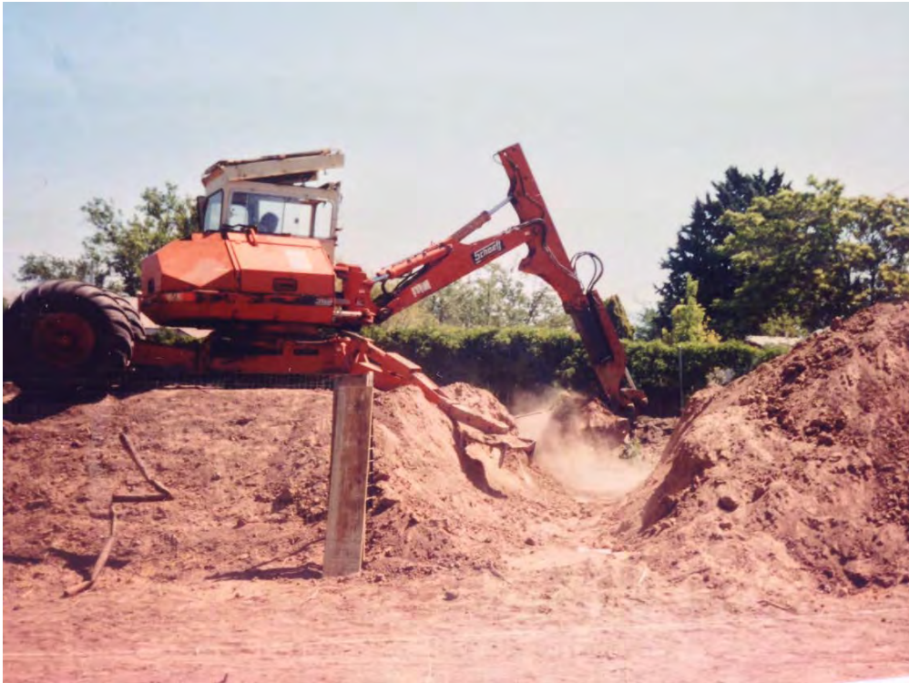
Digging channel for culvert into field
