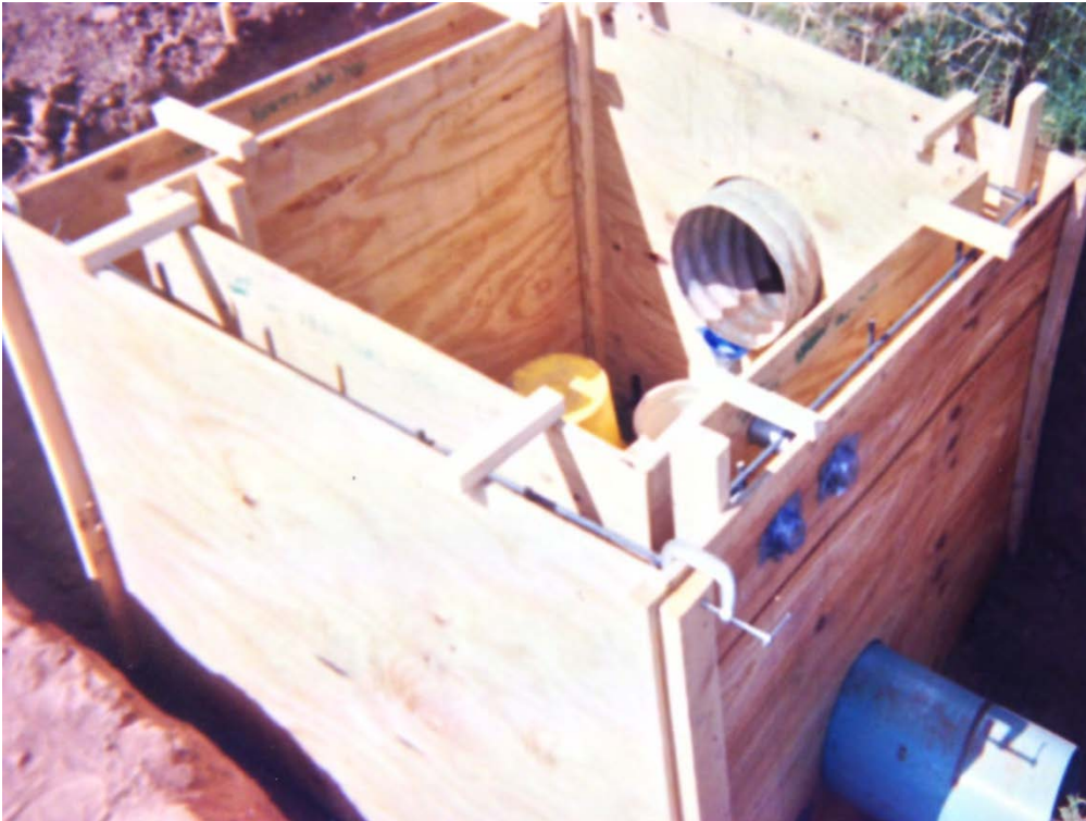
Forming water control structure
